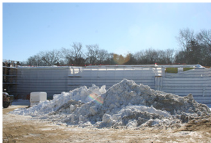
"tent" to allow for exterior brick to be set
