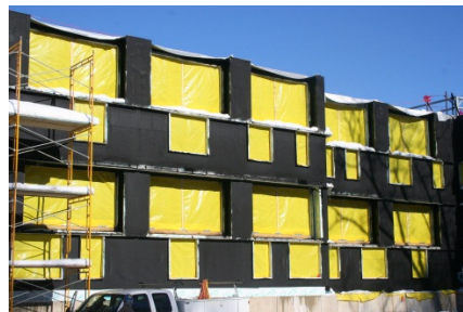
Outside view of 2 floors of classrooms (yellow plastic is temporary windows)
