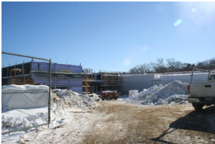
View from School St. of gym & Upper School
