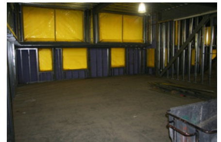
Inside view of typical classroom
