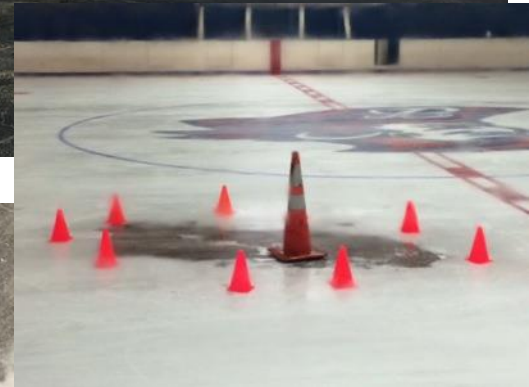
Frost heaves/sub floor failure
